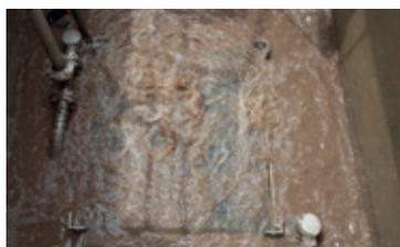
A view inside a tank with an Alfa Laval MBR module treating wastewater from speciality chemicals
